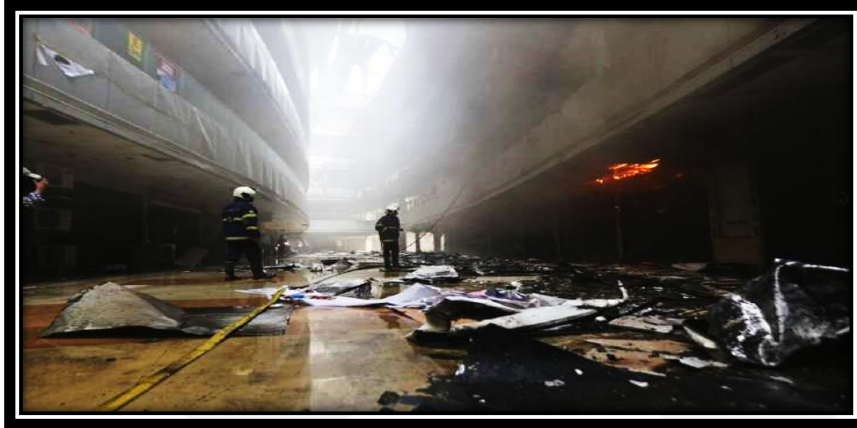
(Fig: Fire fighters trying to douse fire at Sunrise hospital at Bhandup) 15
